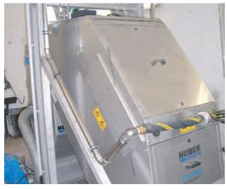
Fully enclosed, odour-free STEP SCREEN® Flexible SSF
