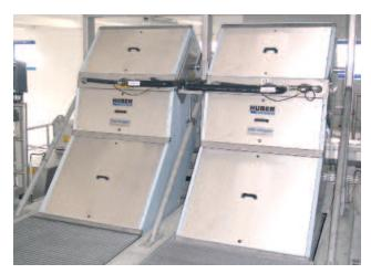
Two STEP SCREEN® Flexible SSF units installed in parallel channels
