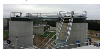
The gas covers were provided with the necessary ancillaries, such as the ballasts, sight port assemblies, sample hatch covers, pressure/vacuum relief valves and emergency relief valves.
